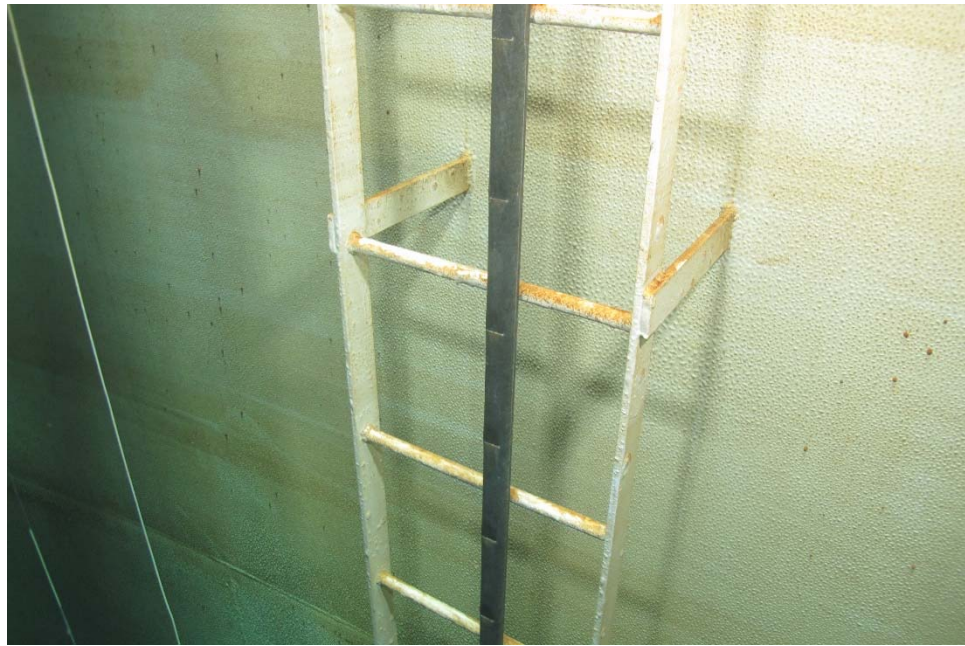
I-29 Same as Photo I-28, except further down the ladder.
