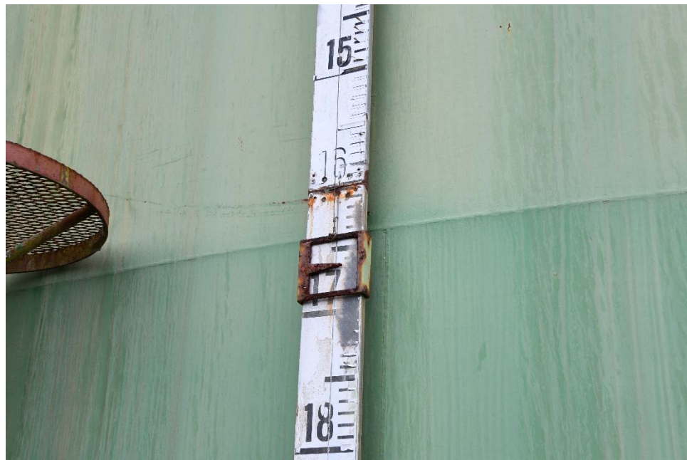
E-23 View of the liquid level indicator gauge board, illustrating the overall poor condition of the gauge board and target.
