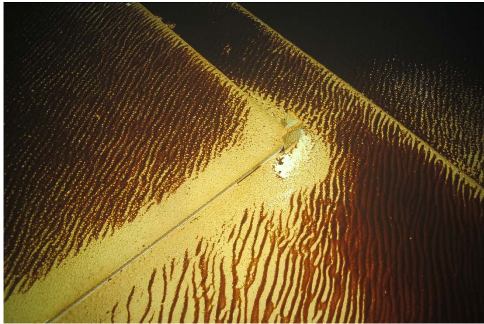
I-44 Same as Photos I-42 and I-43, except a close-up view of a retainer clip. Note blistering on all visible surfaces.
