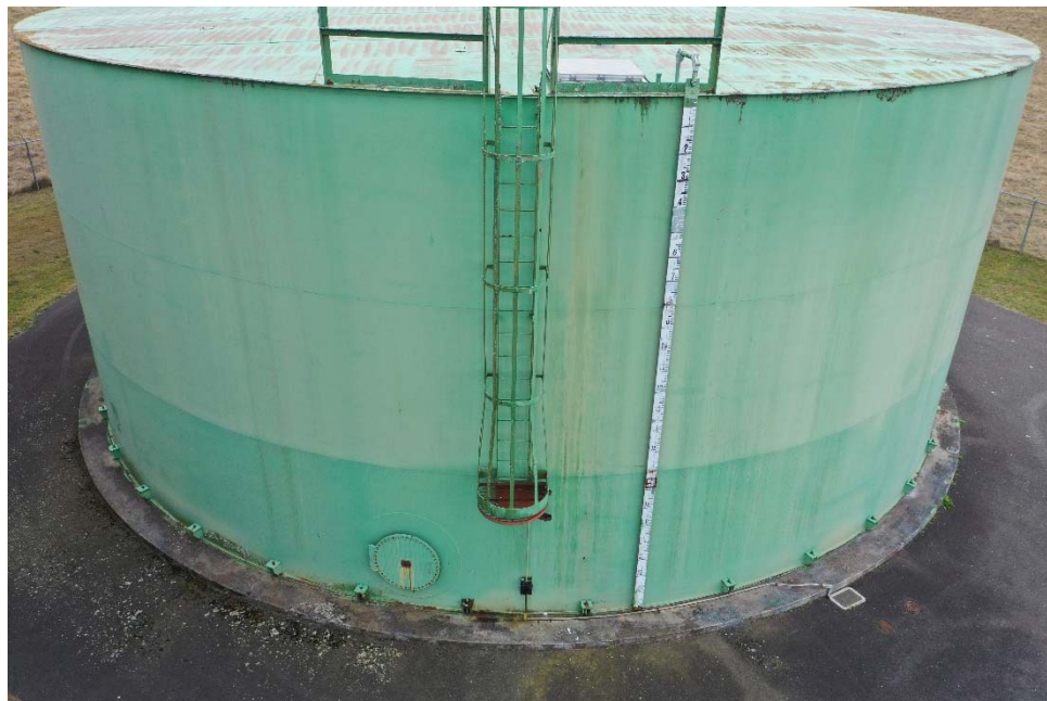
E-14 Same as Photo E-13, except further down the ladder.
