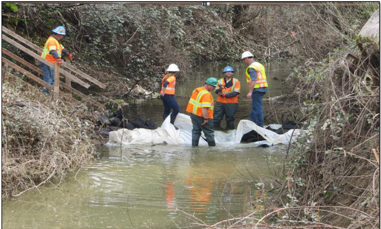
Fish relocation for highway construction at the Willits Bypass project.
