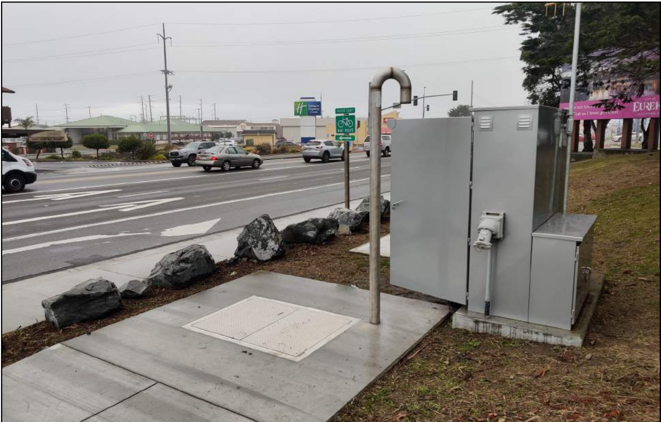
As an on-call consultant to the City of Eureka, SHN provided engineering services for a lift station rehabilitation at the corner of Eureka's Broadway and Del Norte Streets.
