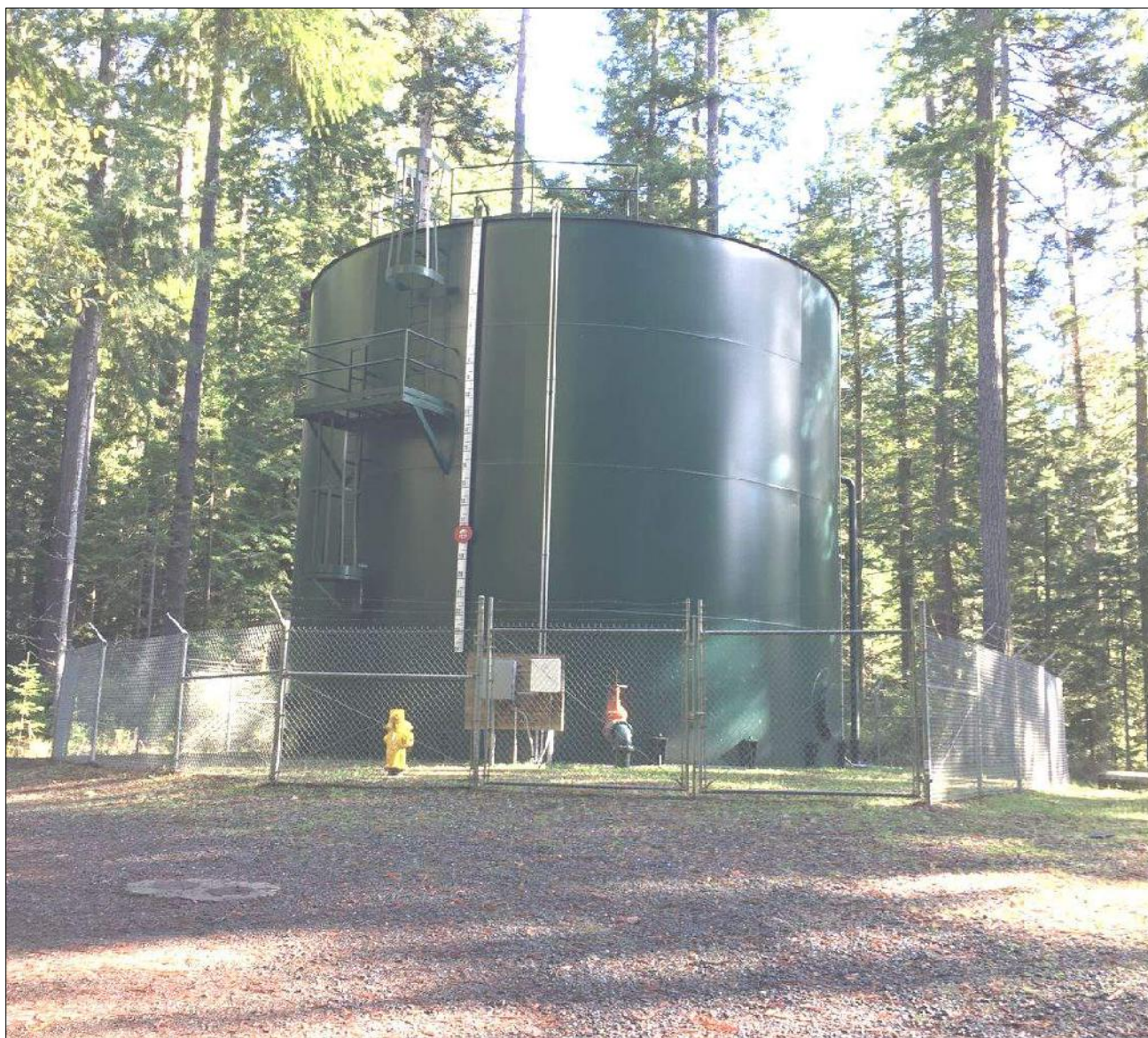
SHN was the project engineer for the City of Arcata's Upper California tank (welded steel).
