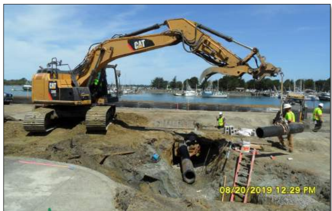
SHN provided construction management services on the City of Eureka's Waterfront Drive project in 2019.
