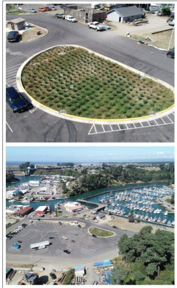
This photo presents a regraded and paved parking area with bioretention swale capturing and treating 100% of paved area runoff. The Noyo Harbor Boat Launch Facilities project was honored with a Merit Award from the American Council of Engineering Companies of California (ACEC).
