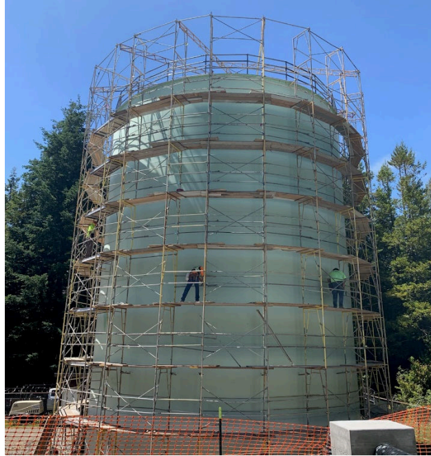
Figure 1: Ridgewood Tank with scaffolding and contractors hard at work.
