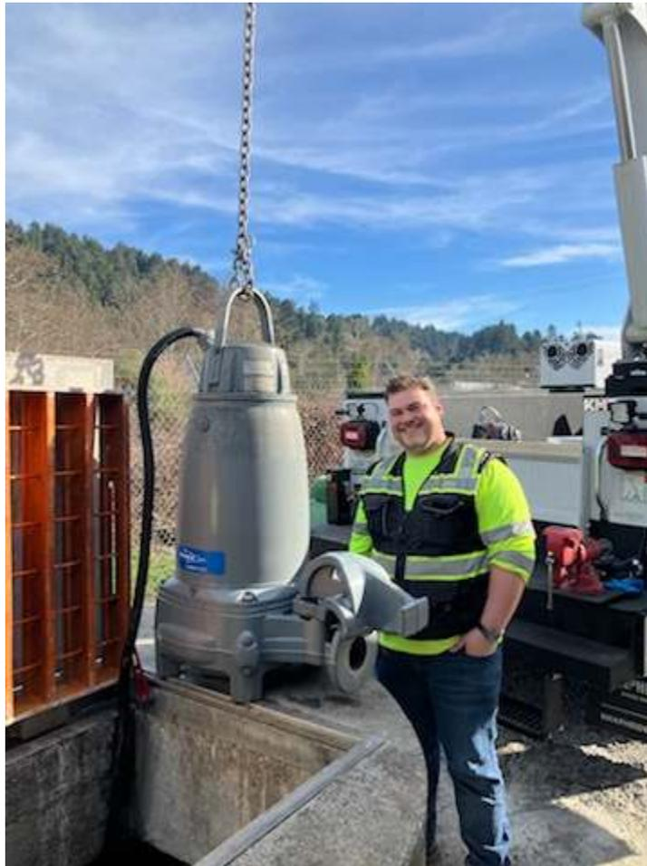
**Figure 1:** This picture shows the 60 HP Pump size comparison to one of our District Staff (Jacob Mitchell) before being installed into the sewer wet well
